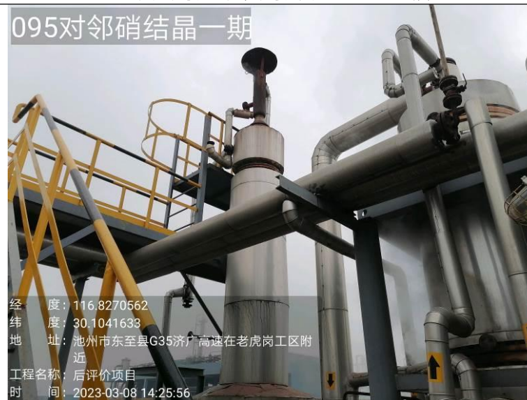
“一级冷凝+间位低油吸收”，DA095 排气筒
